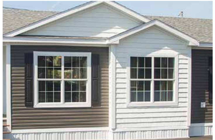
26'-8" Dormer with Bump-Out - Shown with Optional Shake and only Available on 5/12 & Steeper roofs
