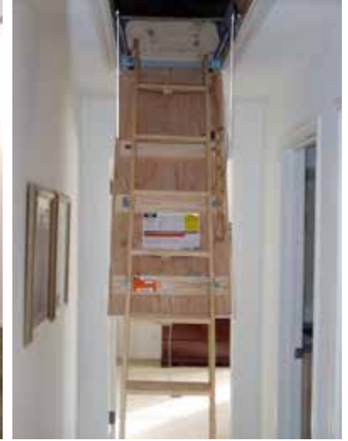
Attic Access with Pull Down Stairs
